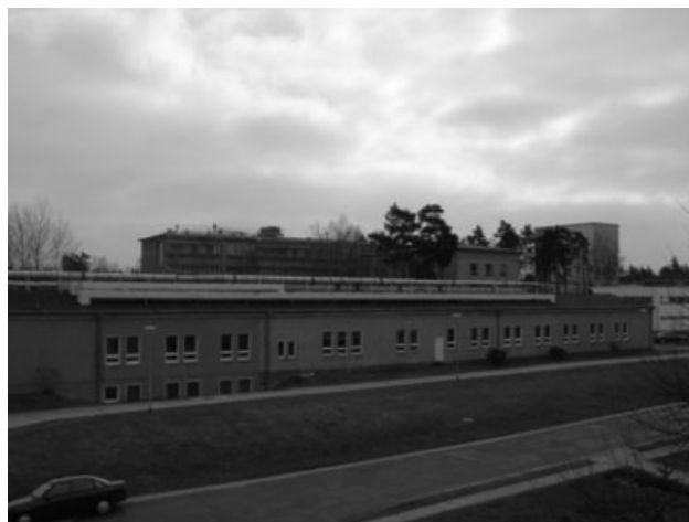
Figure 2 Production building of the Technological Centre.
