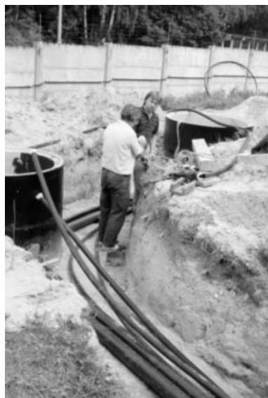
Figure 7 Installation of a transportation system for radioactive gases and fluids.
